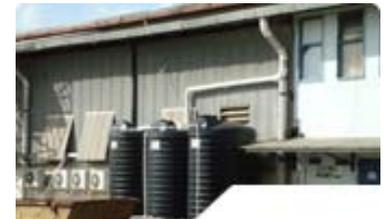
In our Caribbean operations, the team has been finding innovative ways to capture rain water. The Waterloo and Galeota depots both have four 1,000-gallon water tanks to collect rain water run-off. This water is used to flush toilets and damp down the site during dry spells to reduce local dust pollution, which is a problem on these coastal sites.
